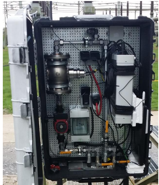
Fig 2 Realization of monitoring system
