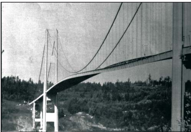
Fig. 1: The swinging Tacoma bridge.
